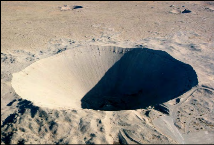
THE " SEDAN " TEST PRODUCED THIS CRATER IT IS 1,280 FT. WIDE AND 320 FT. DEEP.
