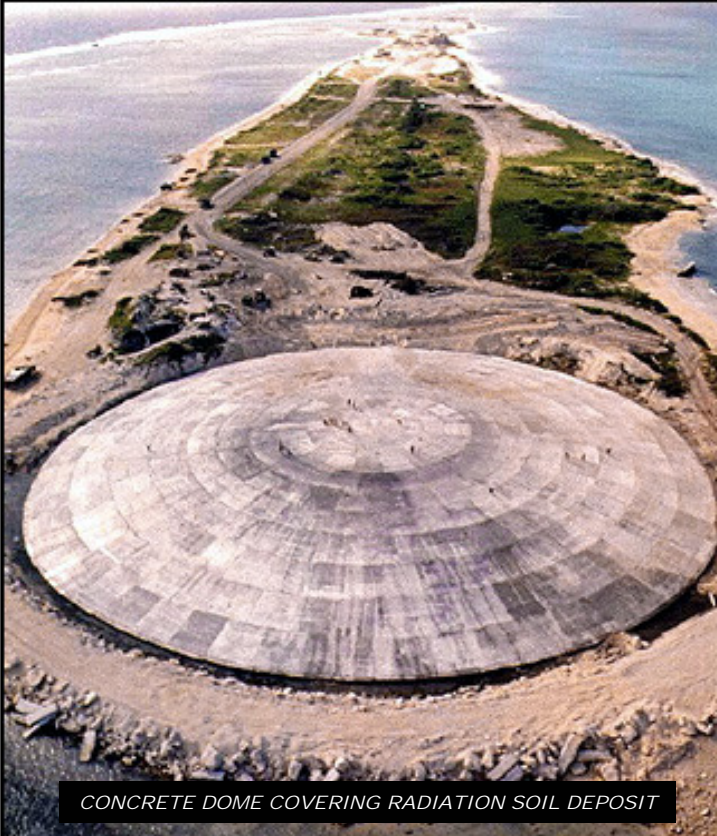
CONCRETE DOME COVERING RADIATION SOIL DEPOSIT
