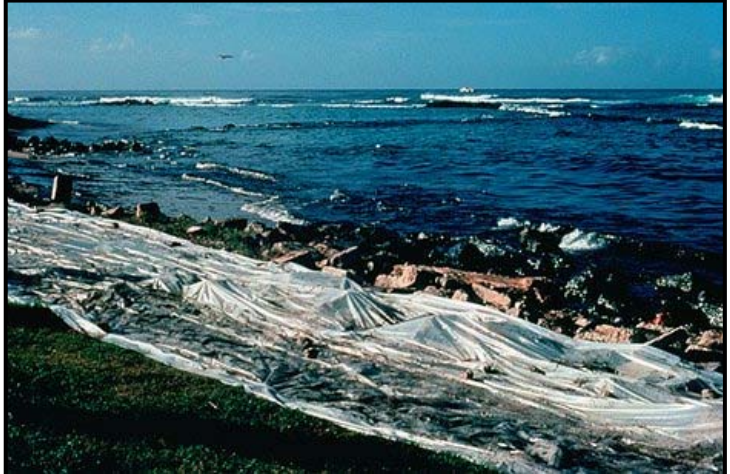
HIGHLY CONTAMINATED SOIL IS MARKED WITH PLASTIC PRIOR TO BEING REMOVED FROM THIS LOCATION
