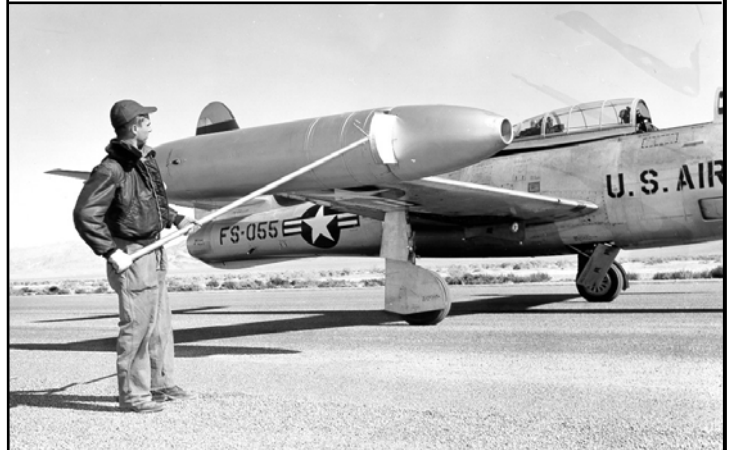
THIS AIR-FORCE GROUND TECH. IS REMOVING RADIATION SAMPLES FROM THE MODIFIED WING-POD OF A CLOUD SAMPLING DRONE AIRCRAFT, AND HE WAS NOT REQUIRED TO WEAR ANY ( RADIATION ) PROTECTION GEAR. ....
