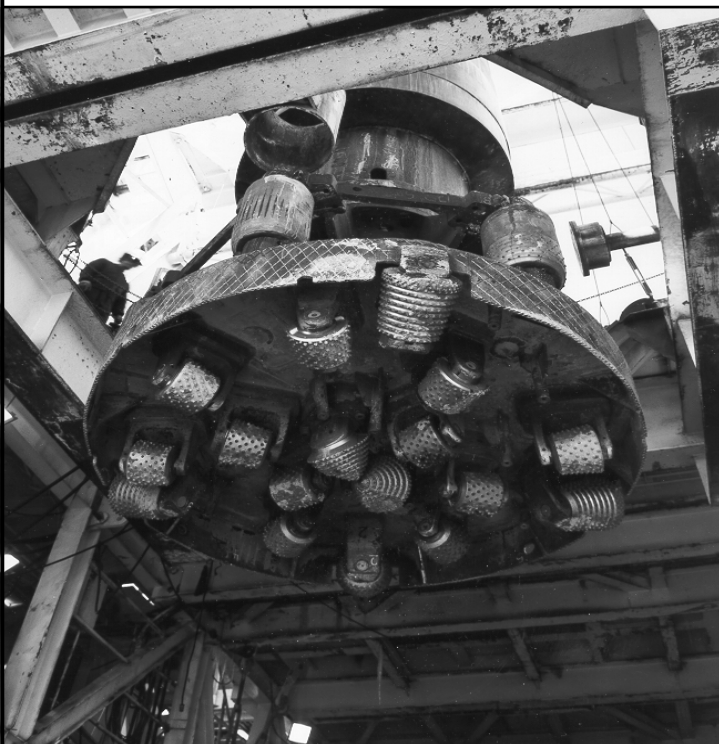
A 60" BIT IS PREPARING TO DRILL A "PRECISION" DEEP SHAFT AT ONE OF THE AMCHITKA TEST SITE LOCATIONS
