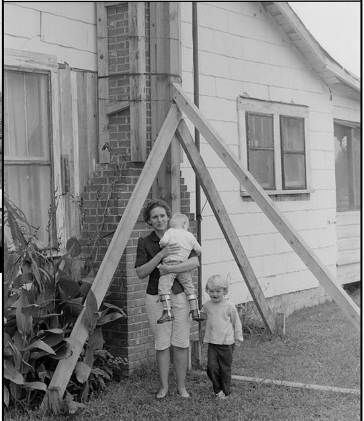
MANY HOMEOWNERS NEAR THE TATUM SALT DOME SITE BRACED THEIR HOMES TO PREVENT DAMAGE PRIOR TO THE TESTS
