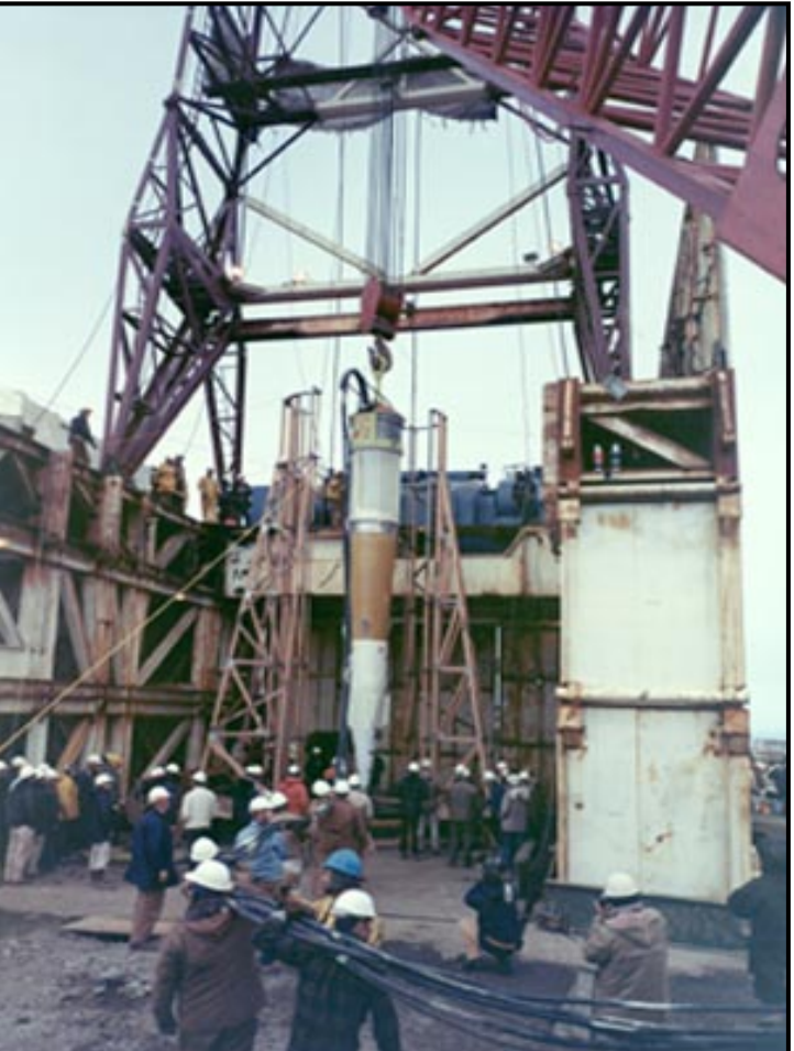
THIS "VELA-UNIFORM" RIG CREW IS PREPARING TO LOWER THE "LONG-SHOT" TEST WEAPON AT THE AMCHITKA TEST SITE
