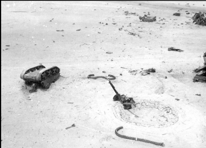
THIS TANK WAS MOVED 400 YDS BY THE ATOMIC TEST BLAST
