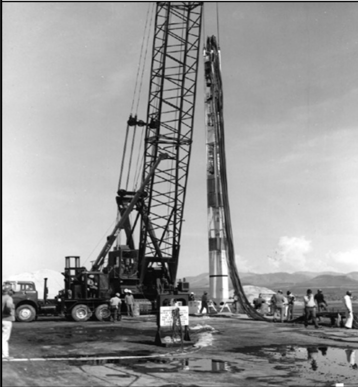
The Nougat "Shrew" device is being lowered into a Yucca-Flats test shaft at the Nevada Test Site on Sept. 16, 1961
