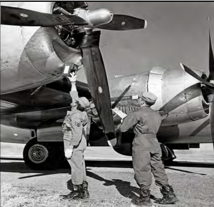
The ( Kwajalein ) ground crew inspects a 'cloud-sampler' aircraft for radiation "hot-spots" after the flight through a nuclear cloud. It is well to note that they are not wearing "radiation" protection suits, or masks while performing those duties . . .
